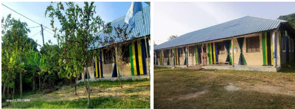
Figure 2: The existing Mahonda Children's Court Building and Site
