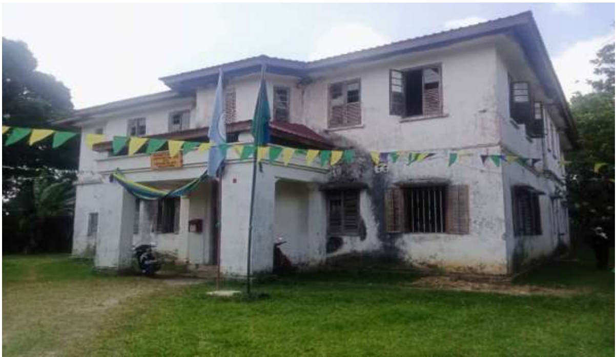
Figure 2: Existing Court Building at Wete
